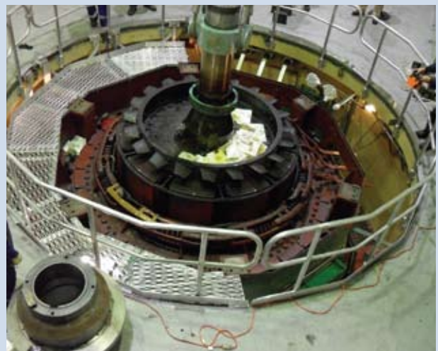
The turbine rotor being lifted out of the generator.
