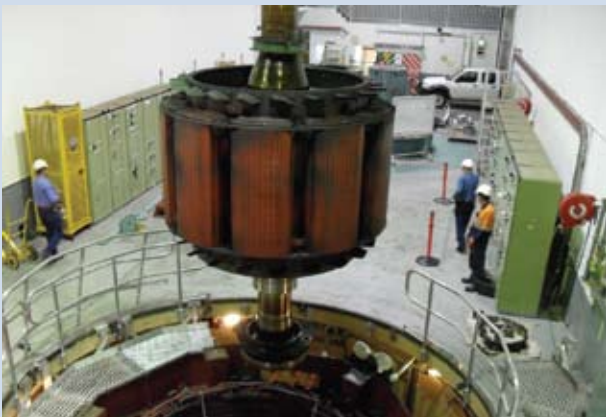
The turbine rotor being lifted out of the generator.
